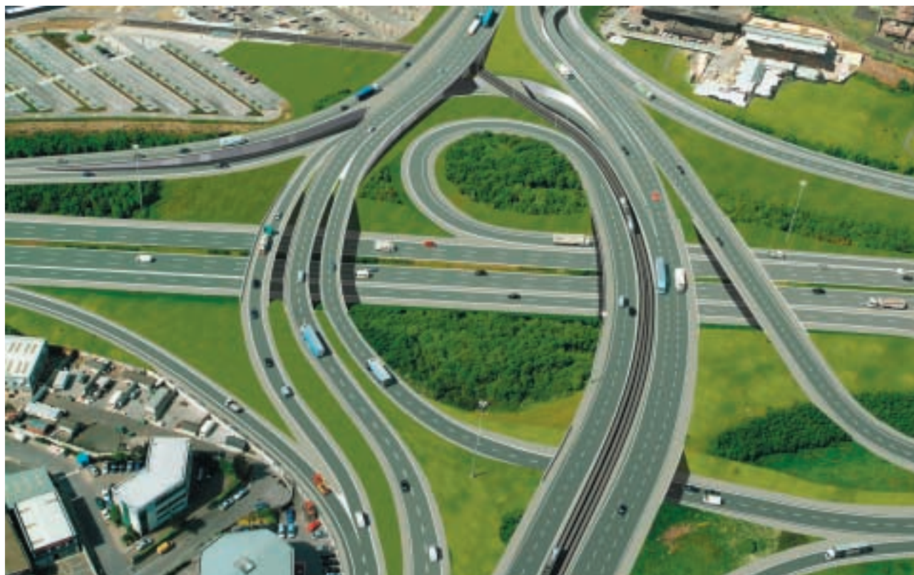
▲ M50 upgrade project a 50/50 joint venture with Ferrovial – M50/N4 interchange
