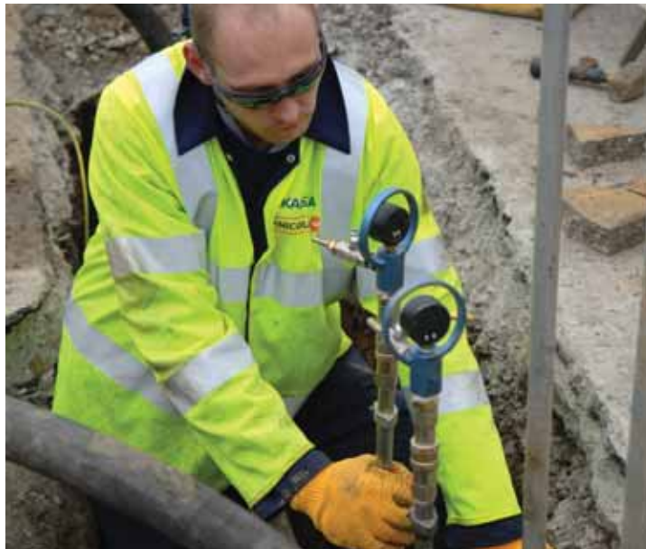
▲ The North London Gas Alliance (NLGA) gas infrastructure replacement project.
